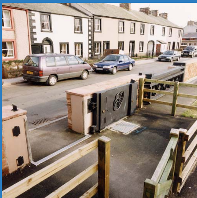
Flood gate to protect properties against flooding.
